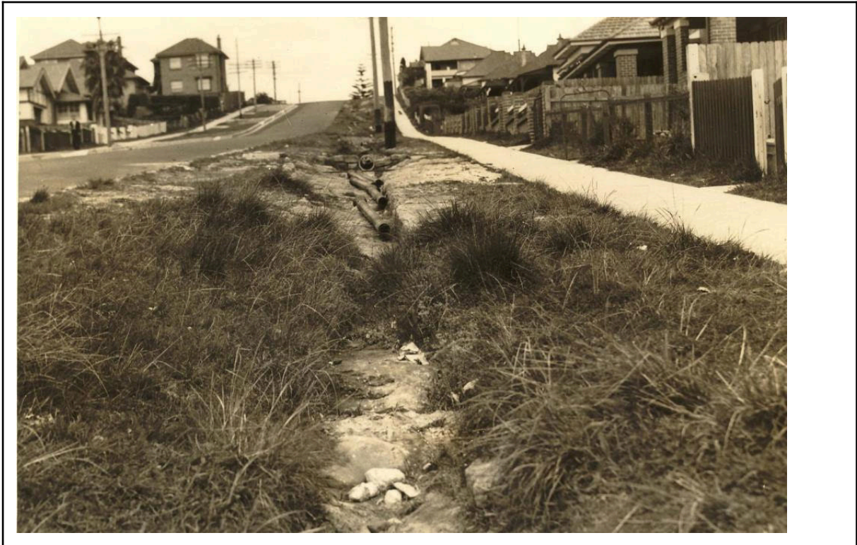
Figure 2 Photograph (14/09/1937) Boyle Street Drain with Unlaid Pipes - Facing upslope
