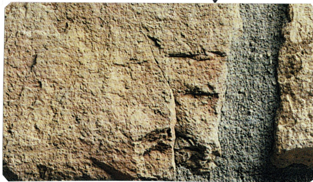
SANDSTONE STEPS AND RETAINING WALLS ↓
