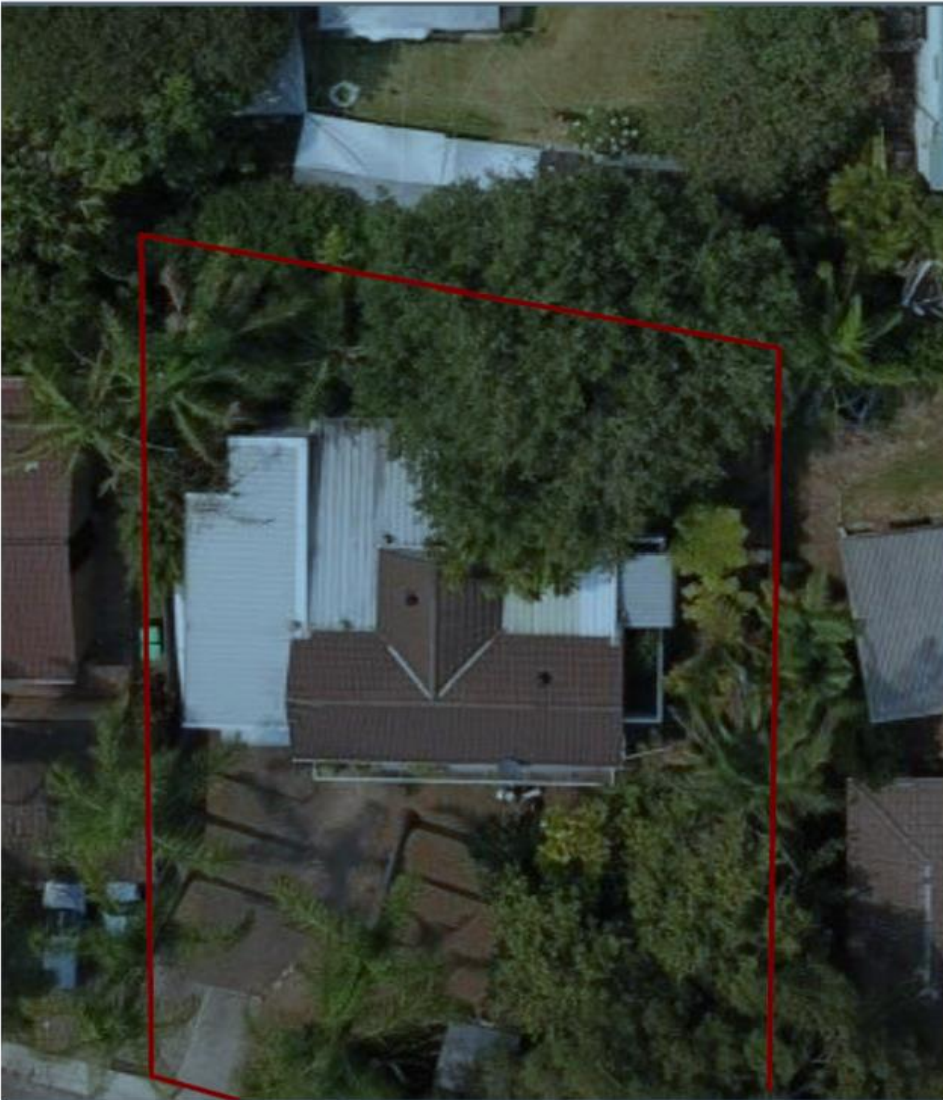
Aerial view of 58 Beaconsfield Street (showing the location of the dwelling and vegetation at the rear)
