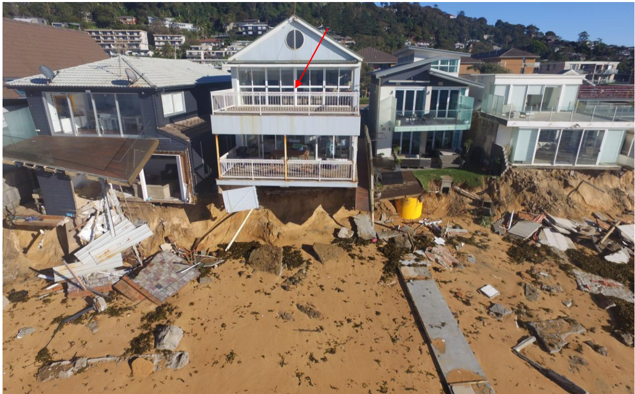
Figure 4: View of coastal storm damage at site on 10 June 2016, with lower balcony evident prior to being demolished, as well as remnants of storage area under the lower balcony
