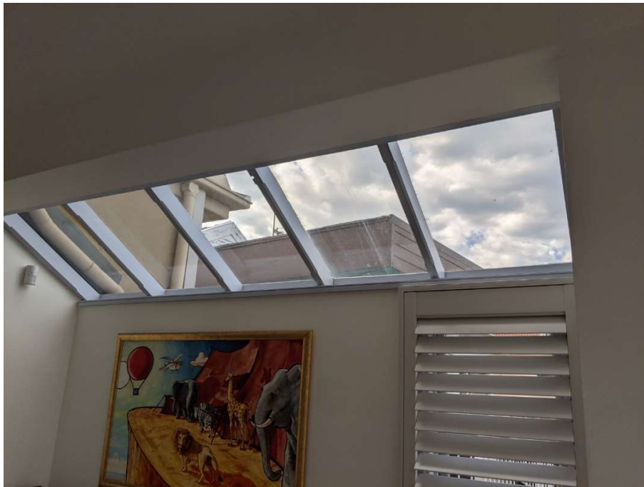
Figure 4: Roof window 14 Addison Road
