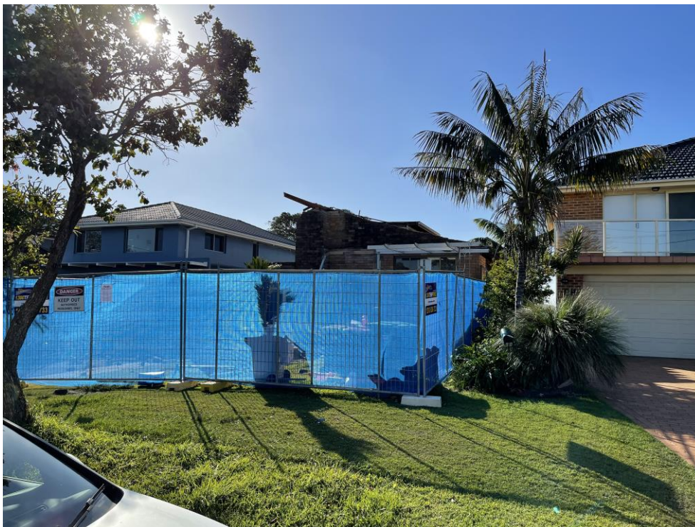
Fig 3: View of the adjoining site to the west at 86 Quirk Street, with new dwelling under construction, looking north-west from Quirk Street
