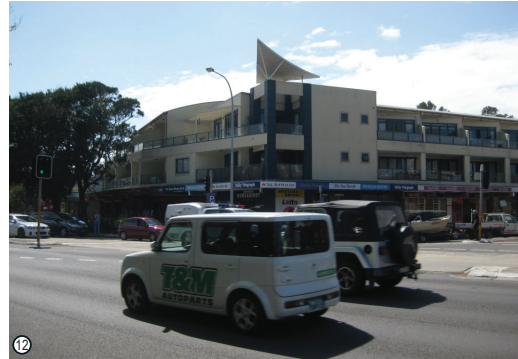
12 Roof articulation on the corner of Pittwater Road and Waterloo Street.
