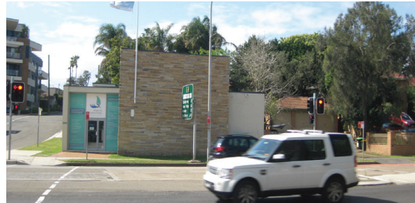
The existing building occupied by Financial Services Company on the corner of Pittwater Road and Albert Street.
