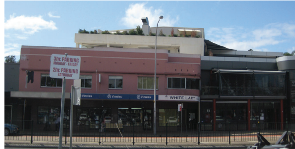
Recent addition to No. 1306 Pittwater Road. Streetwall heights along Pittwater Road varies from 1-3 storeys with taller forms visible beyond the streetwall.
