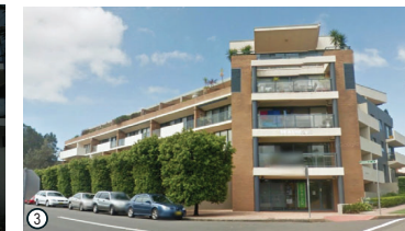
3 5 storeys No. 1-7 Lagoon Street (opposite the site).
