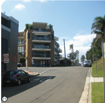
11 5 storey existing building at No. 1-7 Lagoon Street.
