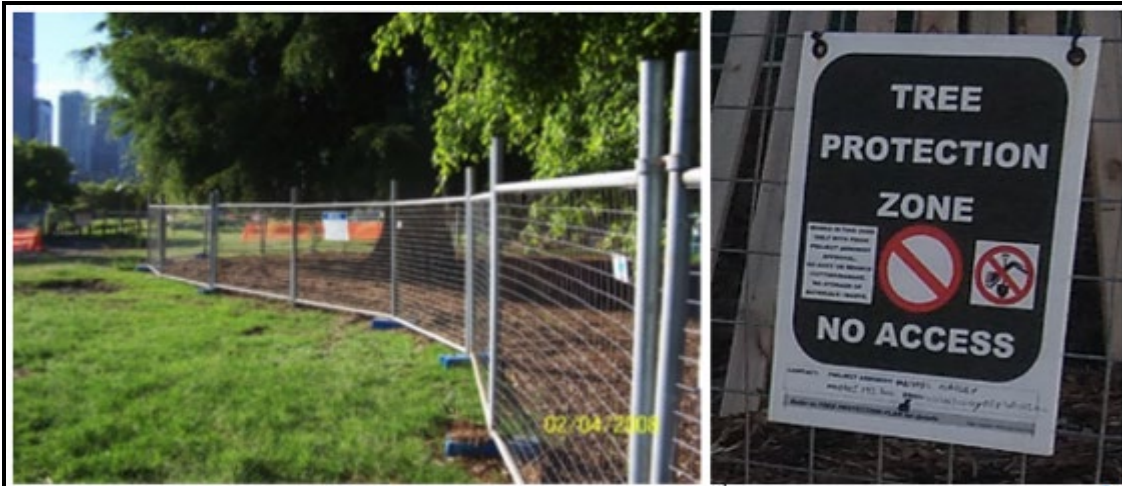
Figure 4. Tree protective fencing and signage.
