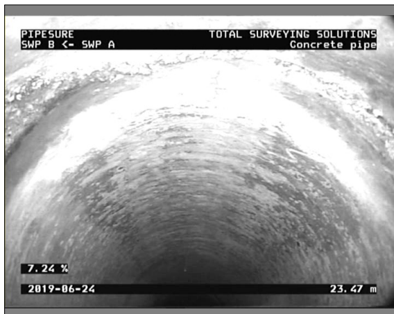
Photo: 1_11A, 00:07:34 23.46m, Infiltration, sweating, at joint , from 12 to 12 o'clock
