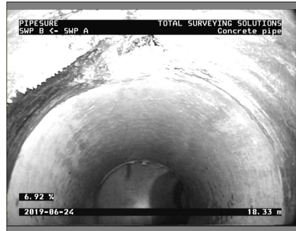
Photo: 1_8A, 00:05:27 18.33m, Spalling of the conduit fabric, localized chipping of one or more of each, at joint , from 12 to 12 o'clock
