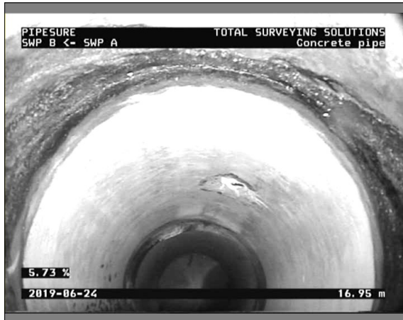
Photo: 1_7A, 00:04:26 16.95m, Infiltration, sweating, at joint , from 12 to 12 o'clock
