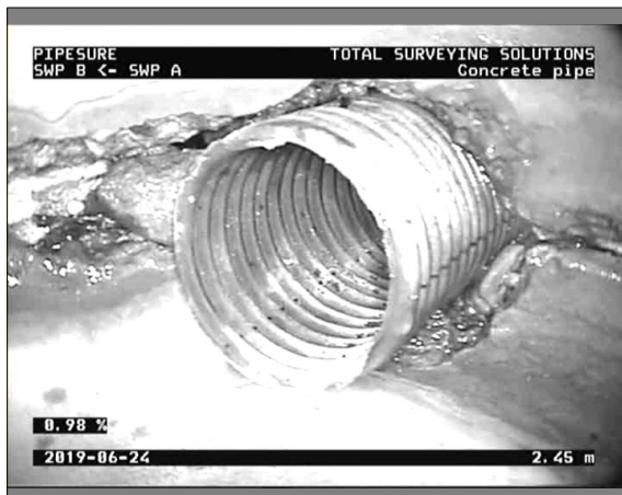
Photo: 1_5A, 00:02:05 2.45m, Junction open, good workmanship, diameter 100mm , General Comments agg line, at 1 o'clock / agg line
