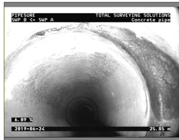
Photo: 1_12A, 00:08:16 25.85m, Infiltration, sweating, at joint , from 1 to 6 o'clock
