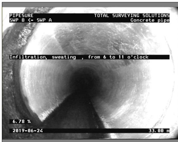
Photo: 1_15A, 00:10:08 33m, Infiltration, sweating , from 6 to 11 o'clock
