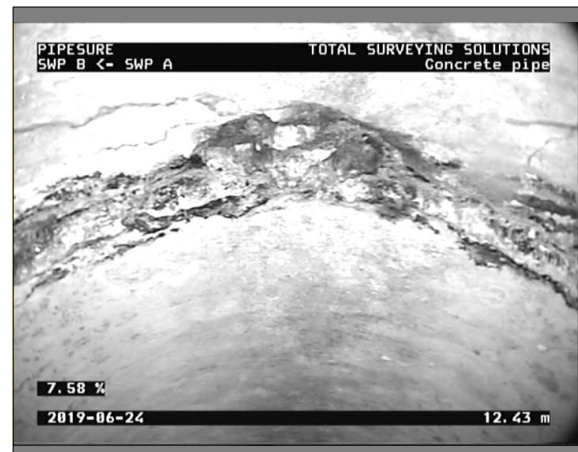
Photo: 1_6A, 00:03:27 12.43m, Spalling of the conduit fabric, localized chipping of one or more of each, at joint , from 12 to 12 o'clock
