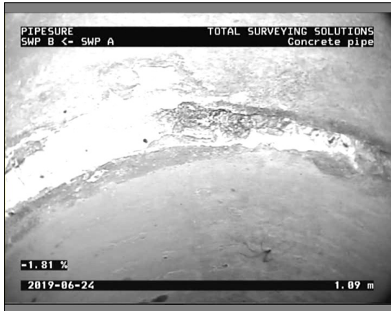
Photo: 1_3A, 00:01:02 1.09m, Joint displaced radially, radial displacement 11-20mm , at 11 o'clock
