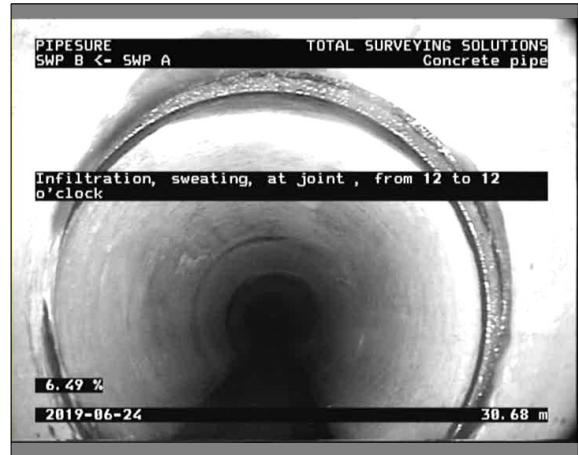
Photo: 1_14A, 00:09:42 30.68m, Infiltration, sweating, at joint , from 12 to 12 o'clock
