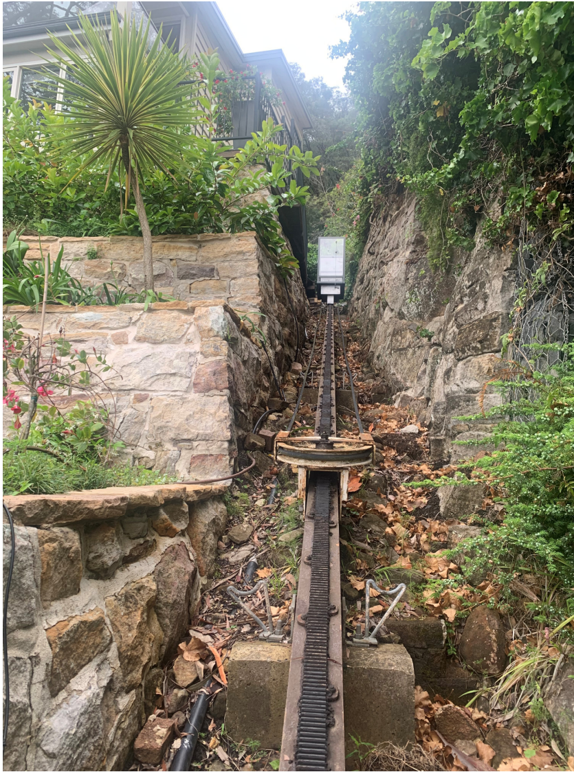
Photo 3 – Standing nearby the lower landing, looking East and along the length of the location of the existing and proposed new lift. In order to accommodate a larger and more comfortable railcar, the proposed new rail is slightly higher off the ground than the existing lift. However, the new rail will still be located substantially below the natural rock wall and existing hedges that sit upon the southern boundary.
