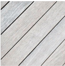
6. Tallow wood timber decking boards to allow to silver naturally
