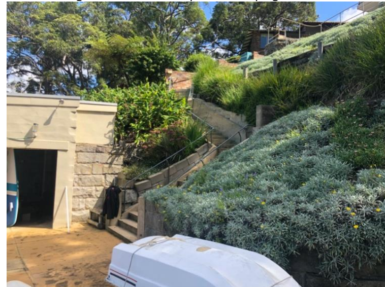
Photo showing uneven steps and poorly constructed retaining walls EXISTING LANDSCAPING
