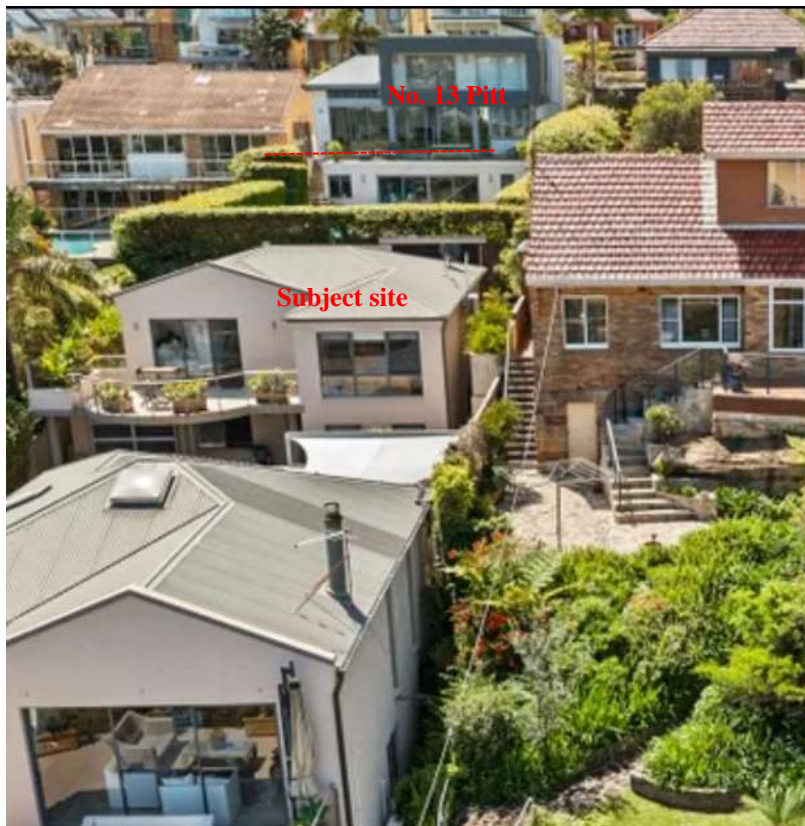
Photo depicting subject site with approx. height and No. 13 Pitt Street
