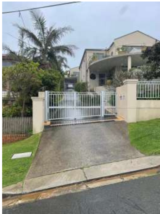
View of Access Handle from Taylor Street (No. 10 Taylor Street in foreground)
