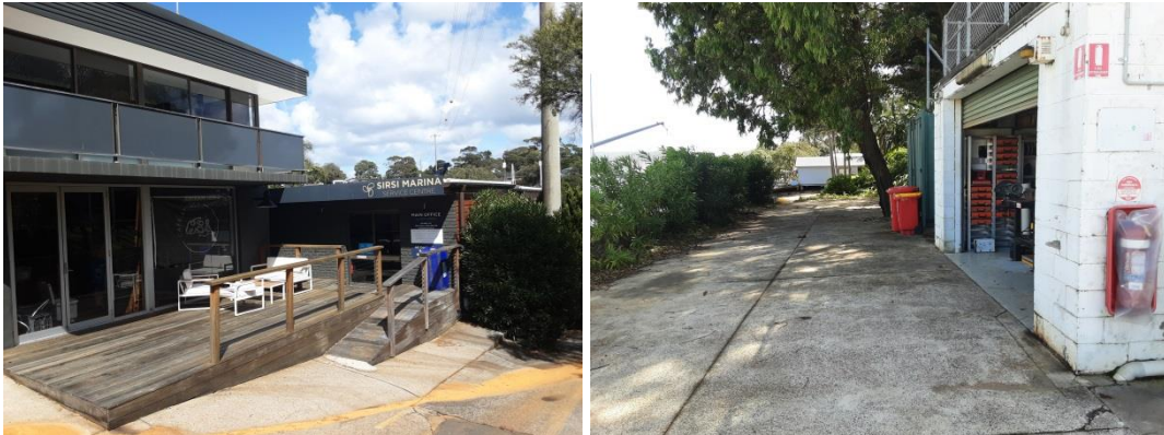
Figures 3-2 and 3-3 showing iron oxide discolouration identified onsite
