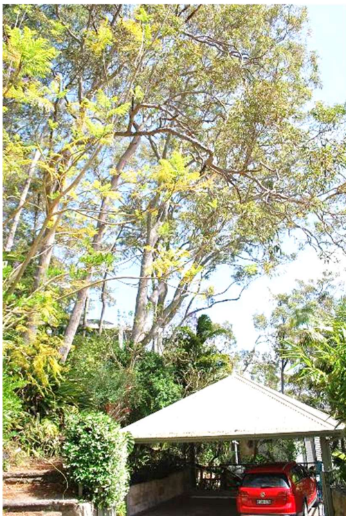
7: Trees P-S and adjacent retaining wall
