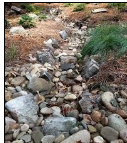
Plate 3 – Low Flow Channel (Australian Wetland Consulting, 2018)
