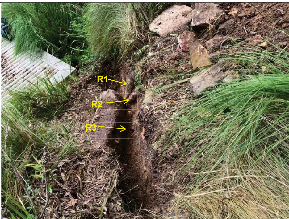
Image 3: Looking North East along root investigation trench 1. Showing location of root 1, 2 and 3.
