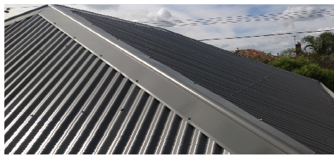
BLUESCOPE STEEL COLOURBOND CUSTOMORB ROOF SHEETING AND CAPPINGS. COLOUR TO COMPLY WITH BCA CLASSIFICATION OF DARK (SOLAR ABSORPTANCE 0.475 - 0.70)
