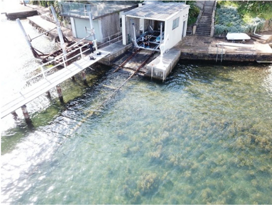
Figure 3 Oblique, low drone view showing concrete ramp plus slipway and boat cradle extending into the boatshed, the block sandstone seawalls and concrete plus sandstone flagged reclamations at the property.
