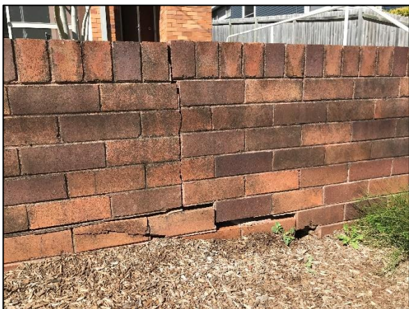
Photograph 9: Cracking in brick retaining wall within front of property
