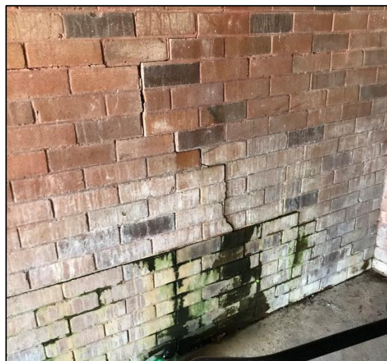
Photograph 8: Moisture and cracking within east wall of garage.
