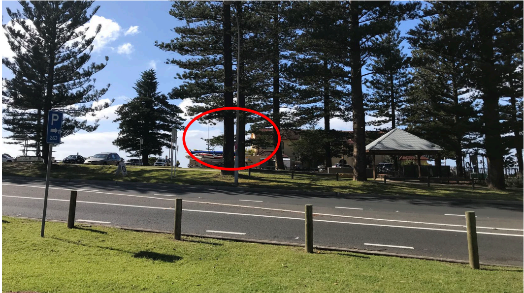
Figure 18 View from western side of Barrenjoey Road, adjacent to 399 Barrenjoey Road. The location of the proposed addition is identified by a red circle (September 2020)
