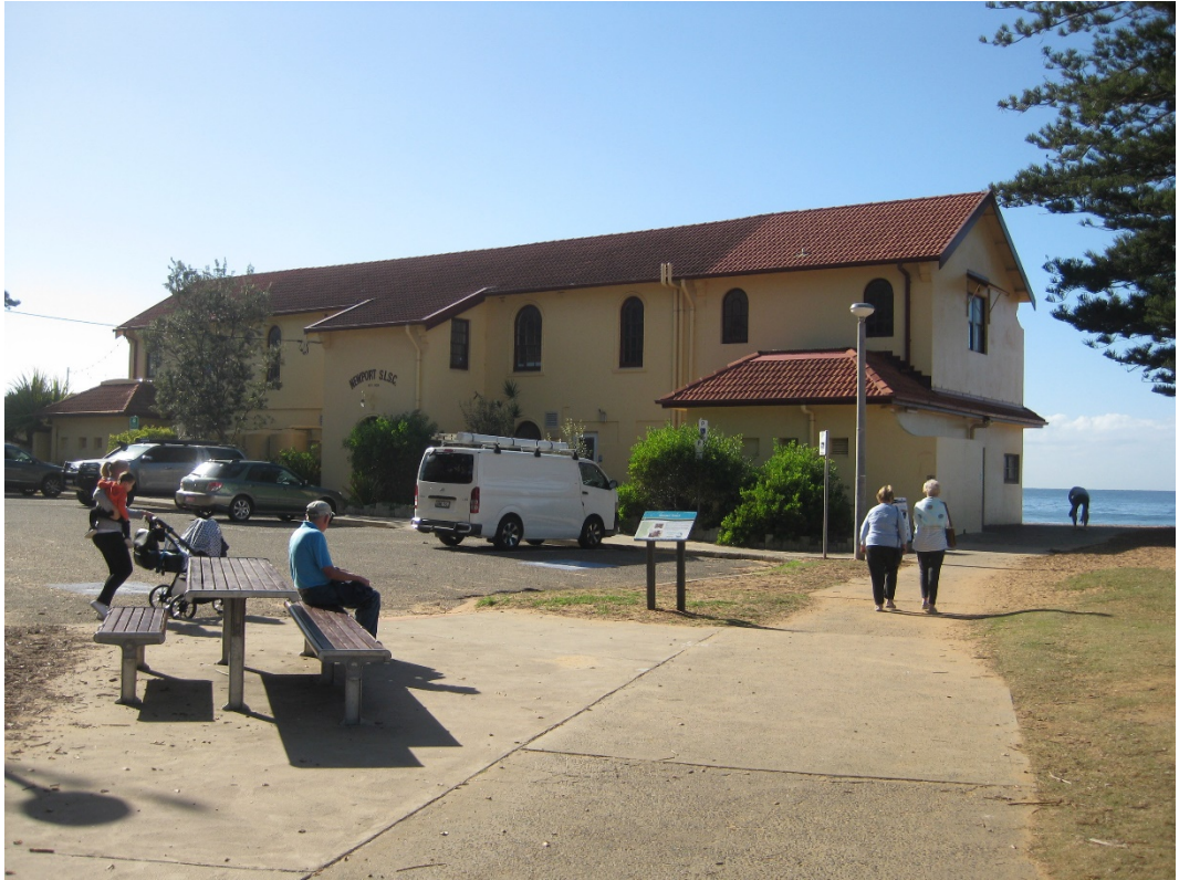
Figure 4 View of the western elevation of Newport SLSC from Bert Payne Park (September 2020)
