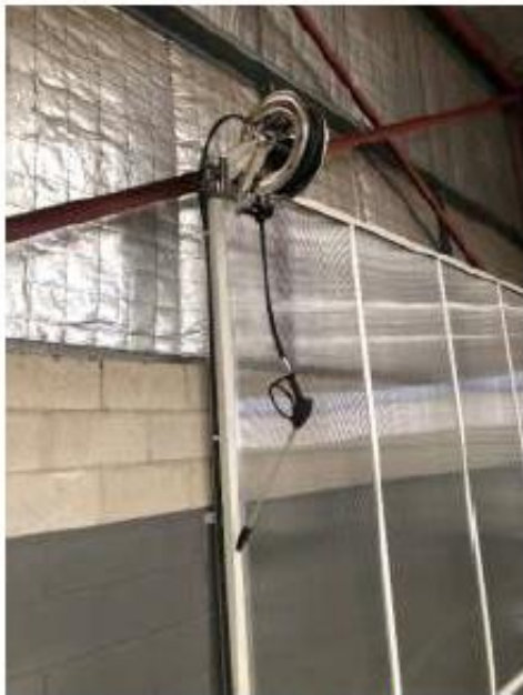
Example of Water Reel and pressure washers
