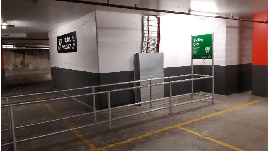
View of the existing trolley bay to be relocated
