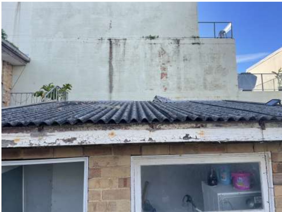
Photograph 4: Image of the suspected corrugated ACM roof of the detached laundry on Lot 2 DP 314645 (photographed 9/6/2023).
