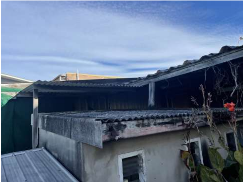
Photograph 13: Image of suspected ACM roofing on the north-western shed at Lot 3 DP 6777.
