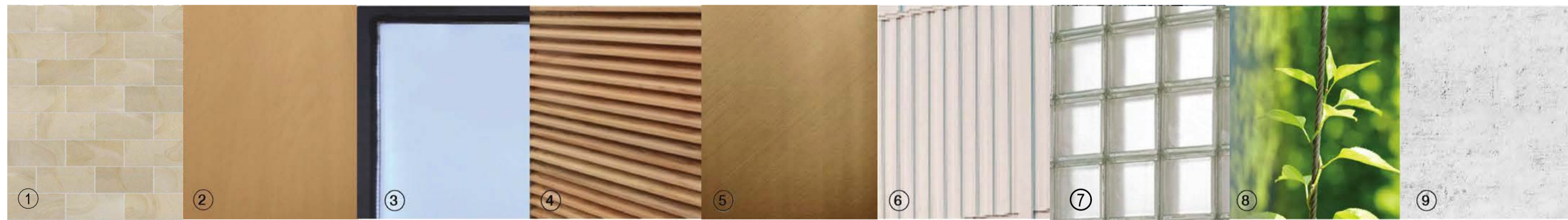
1 Sandstone cladding 2 Render in timber colour 3 Clear glazing & dark metal mullions 4 External venetian louvres 5 Render in bronze colour 6 Light coloured profiled metal 7 Glass blocks 8 Landscaped roof and Ground 9 Smooth concrete
