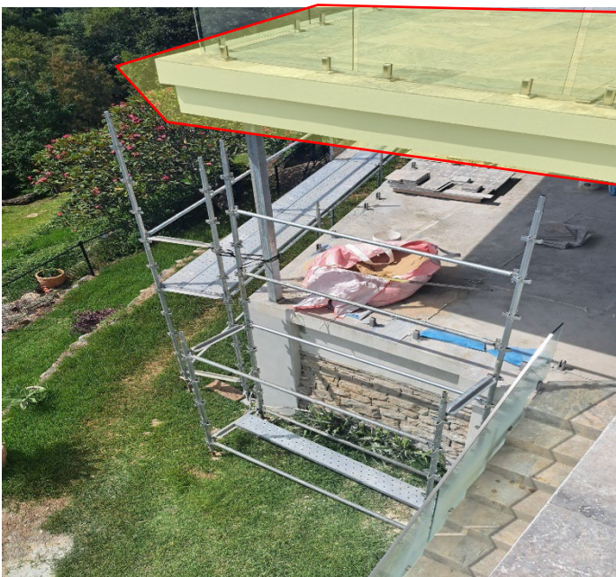
Figure 21 The extended balcony on the second floor outlined in yellow, built above the approved footings and enclosed terrace area of the first floor (source: Gyde)
