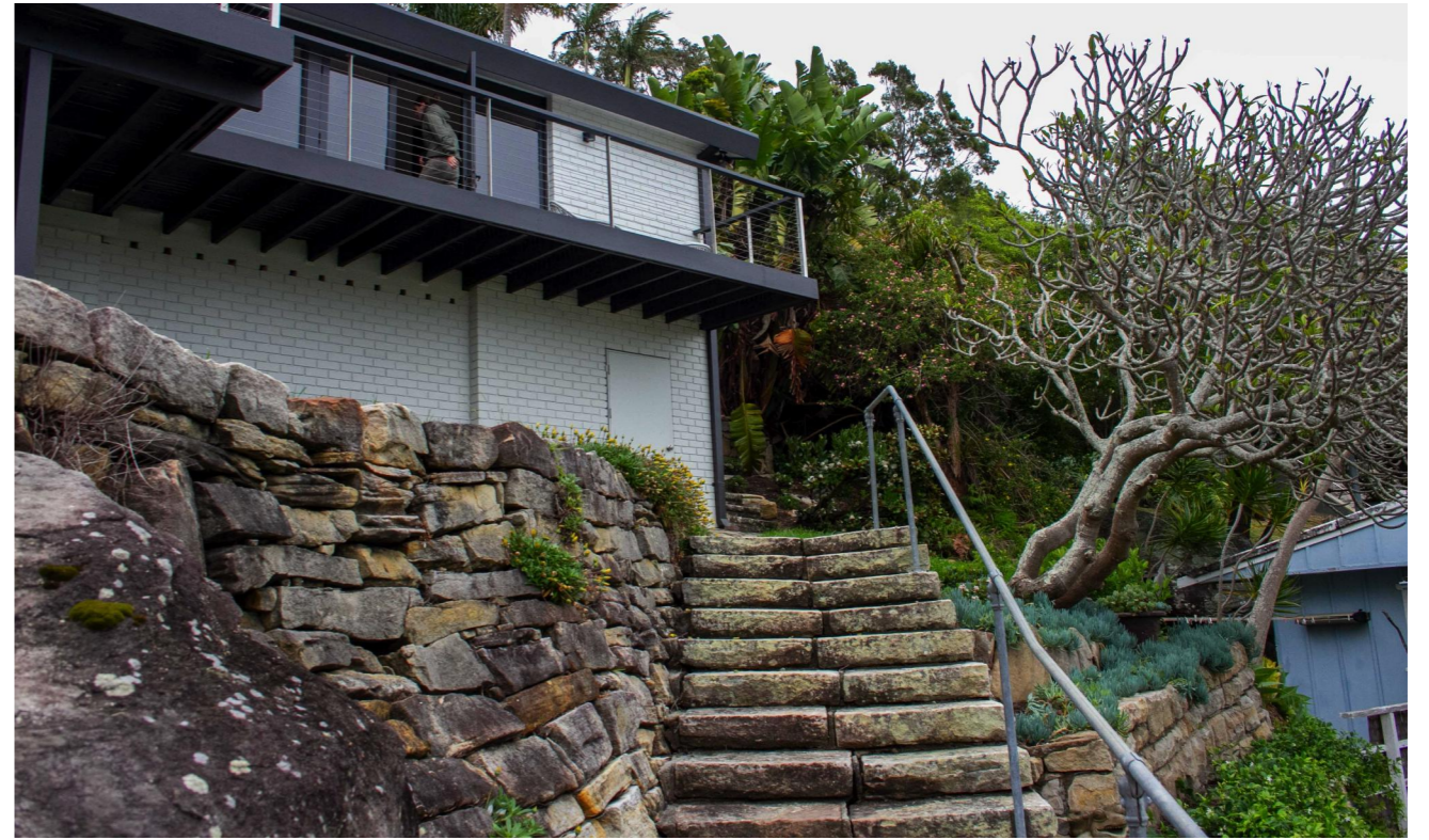
2. EXISTING STAIR ACCESS
