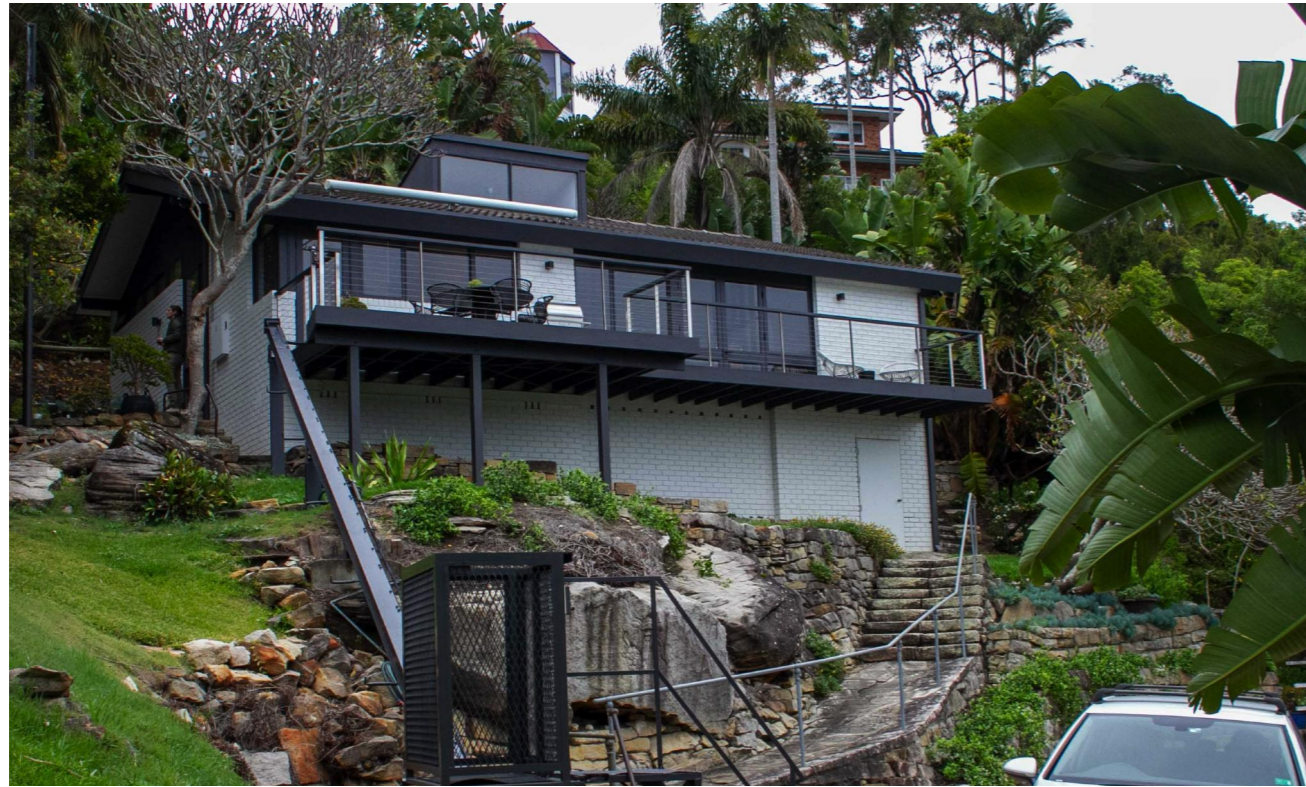
1. EXISTING DWELLING AS VIEWED FROM NORTH
