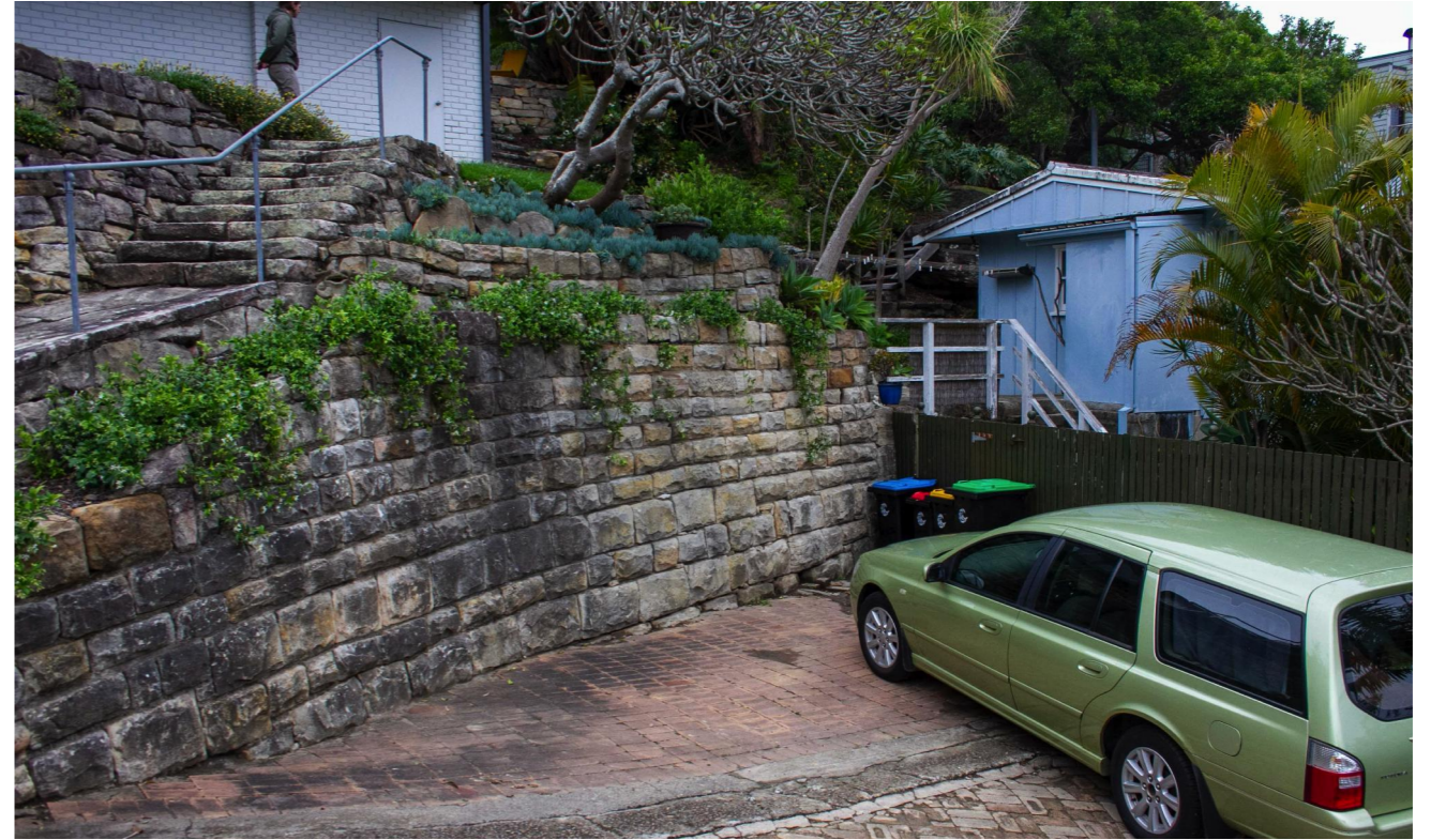
2. REAR OF DRIVEWAY
