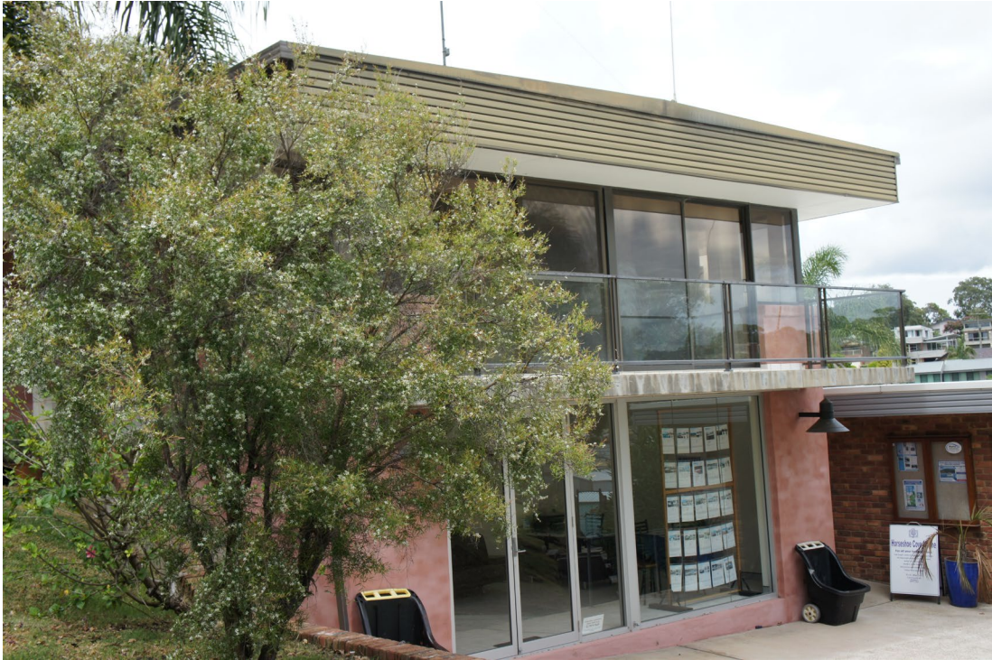
Figure 5: Existing office from marina access road (Scott Carver)
