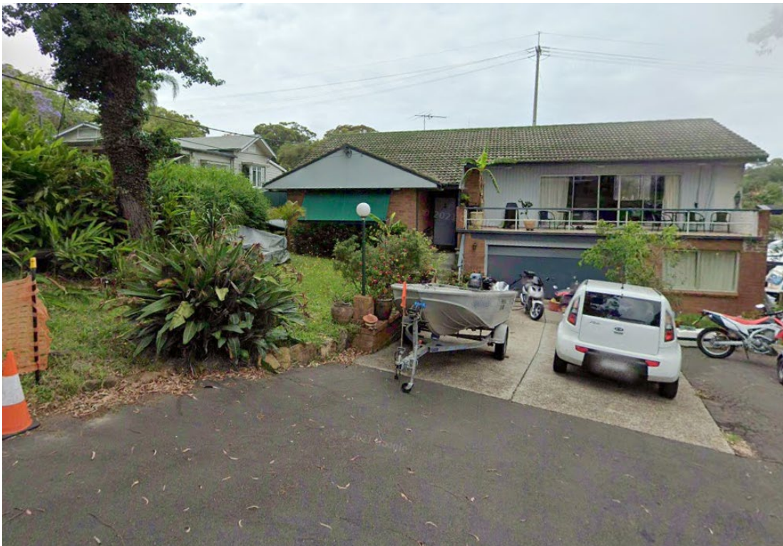
Figure 6: Existing residence at 57 The Avenue, Newport with 55 The Avenue in the background (Google Maps)
