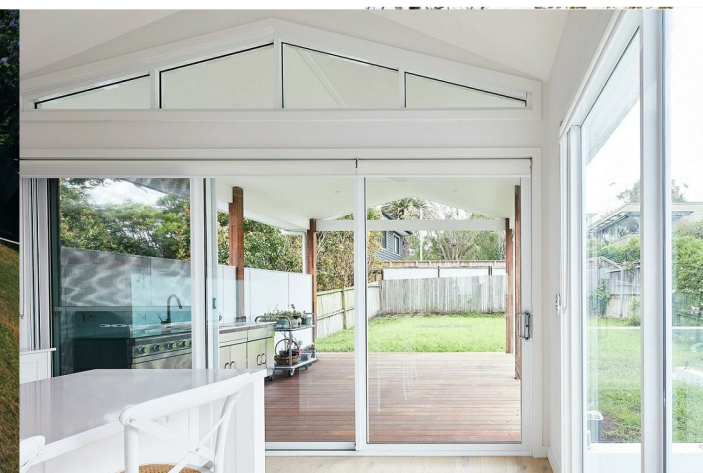
AL1 - Powdercoated aluminium windows and doors
