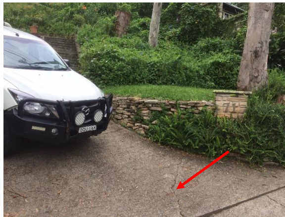
Series-4: Signs of movement in and around the Property
