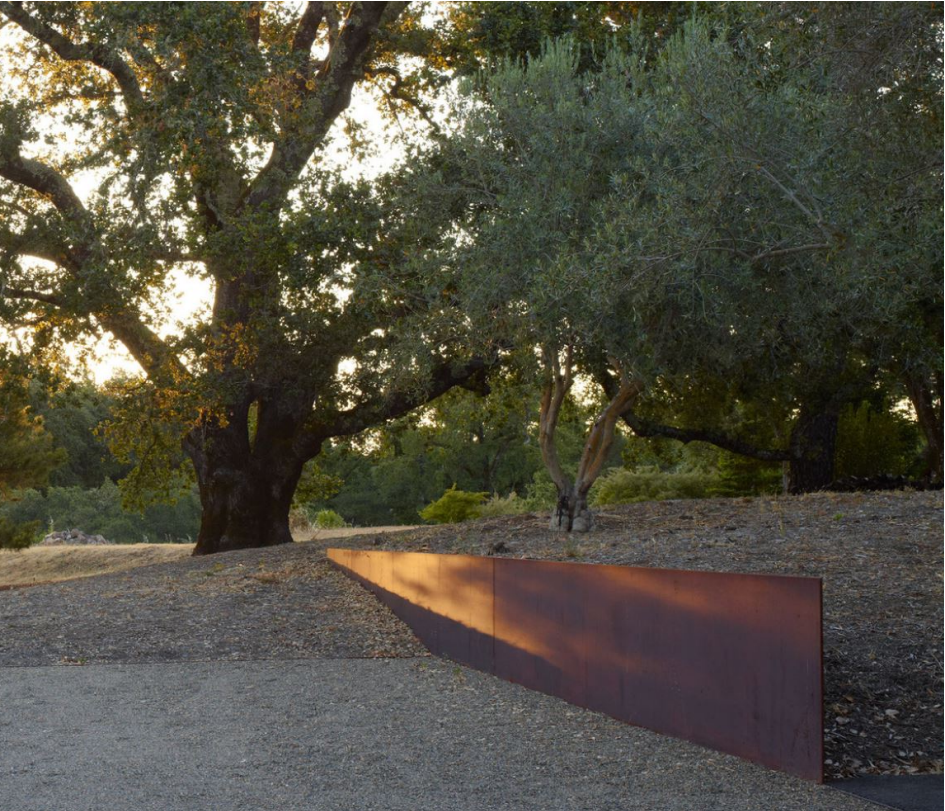
Steel Retaining Walls
