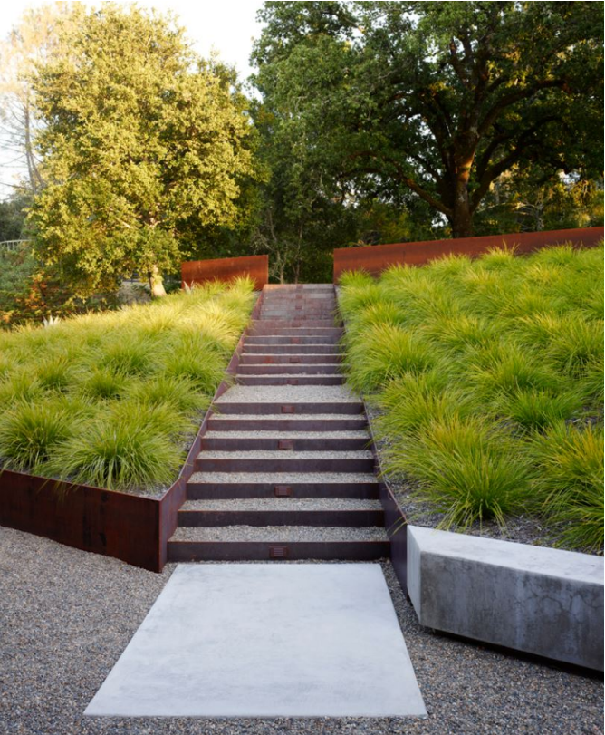
Steel Edging & Finished Concrete
