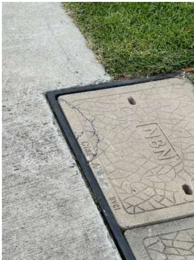
Figure 30 – Crack is evident to the pit outside 13 Bubalo Street Warriewood.
