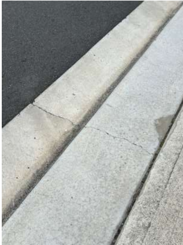
Figure 53 – Crack is evident to the layback outside 3 Bubalo Street Warriewood.
