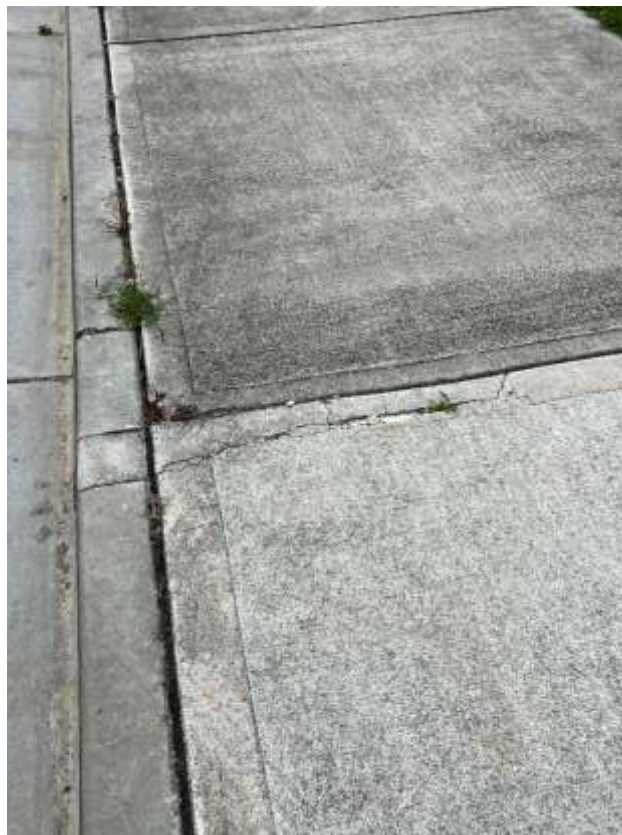
Figure 18 – Crack is evident to the footpath outside 19 Bubalo Street Warriewood.
