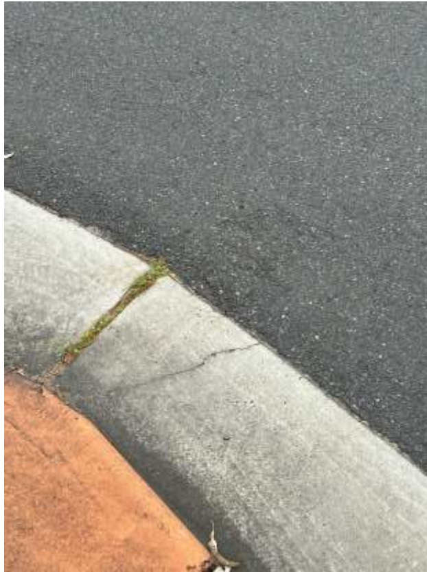
Figure 75 – Crack is evident to the layback outside 61 Warriewood Road Warriewood.
