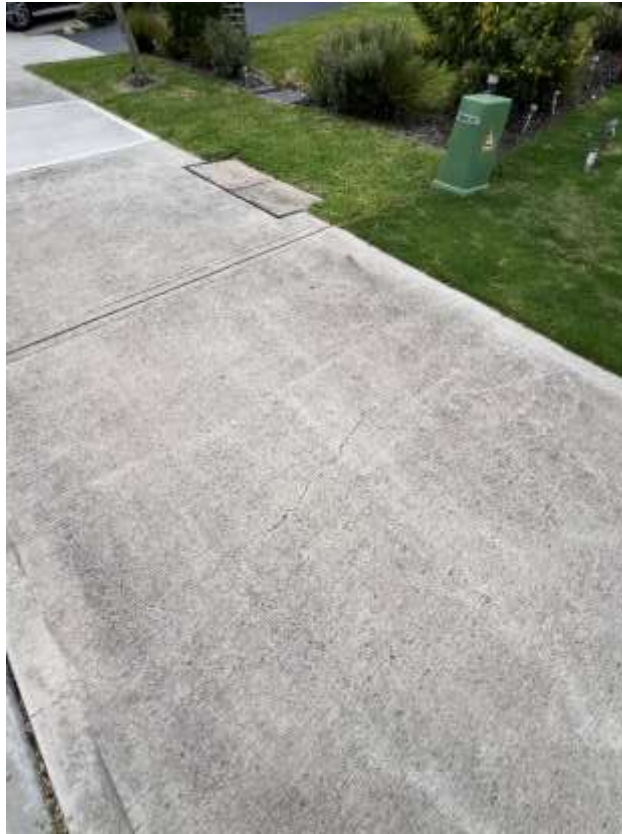
Figure 31 – Crack is evident to the footpath outside 13 Bubalo Street Warriewood.
