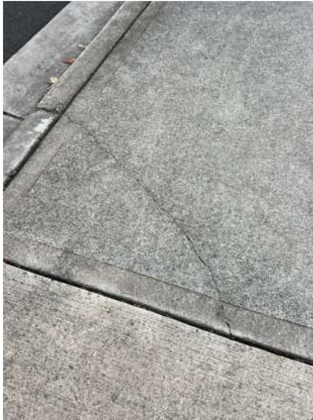
Figure 65 – Crack is evident to the footpath outside 61 Warriewood Road Warriewood.
