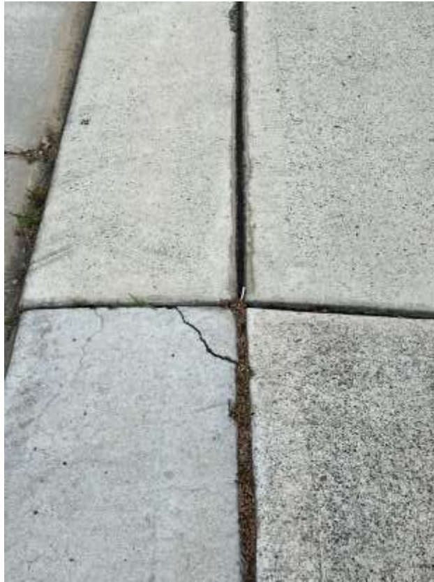
Figure 121 – Crack is evident to the layback outside 18 Bubalo Street Warriewood.
