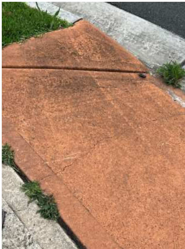
Figure 80 – Crack is evident to the layback outside 63 Warriewood Road Warriewood.
