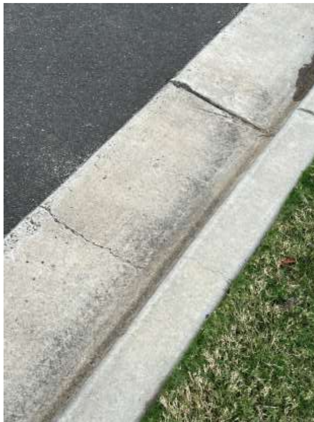
Figure 114 – Crack is evident to the kerb outside 16 Bubalo Street Warriewood.
