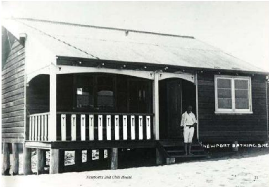
Figure 8. The Club Building in 1915 Source: (Jennings 2009:21)
