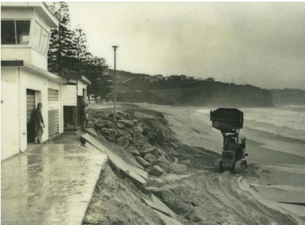
Figure 11. Rock Protection being placed seaward of the Club Building on 28 th May 1974 following a storm Source: (Jennings 2009)
