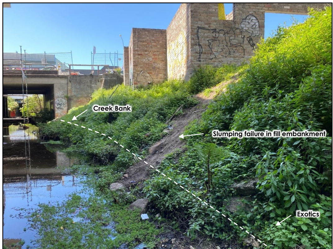
Figure 15: Fill embankment failure with the Site (28/9/2020).
