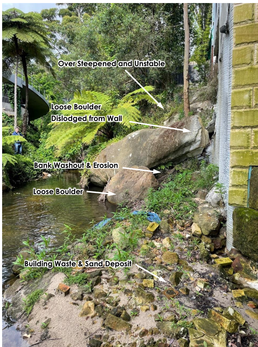
Figure 20: Northern Creek bank and embankment showing failure (17/11/2021).
