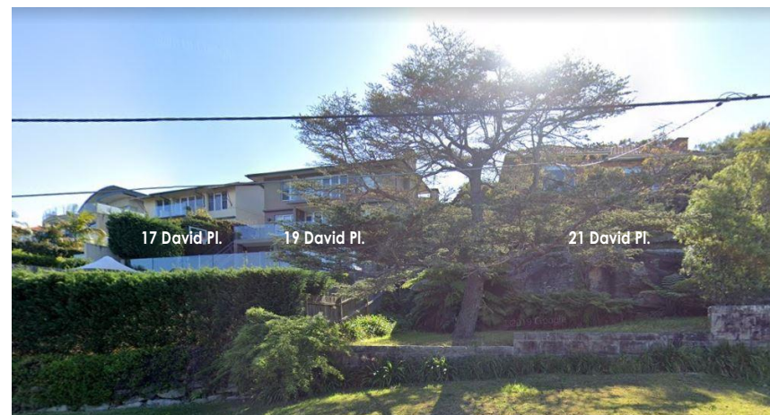
View from Richmond Rd.
