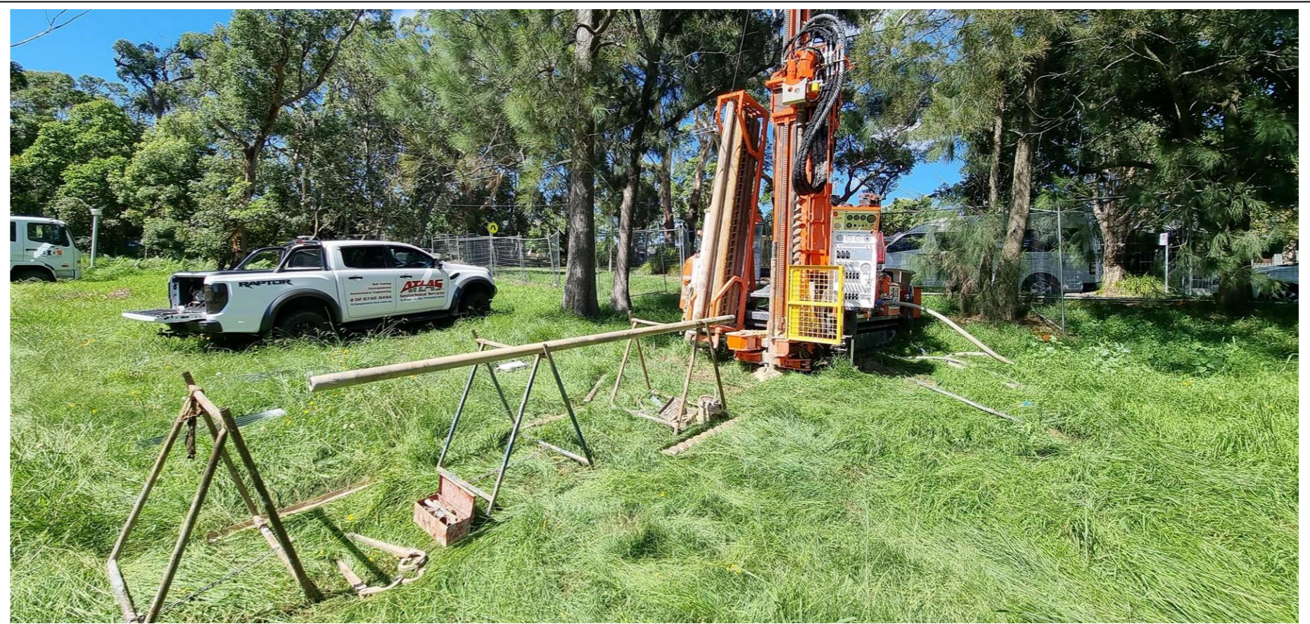
Figure 2.2 – General View of Drilling Operation (BH02)
