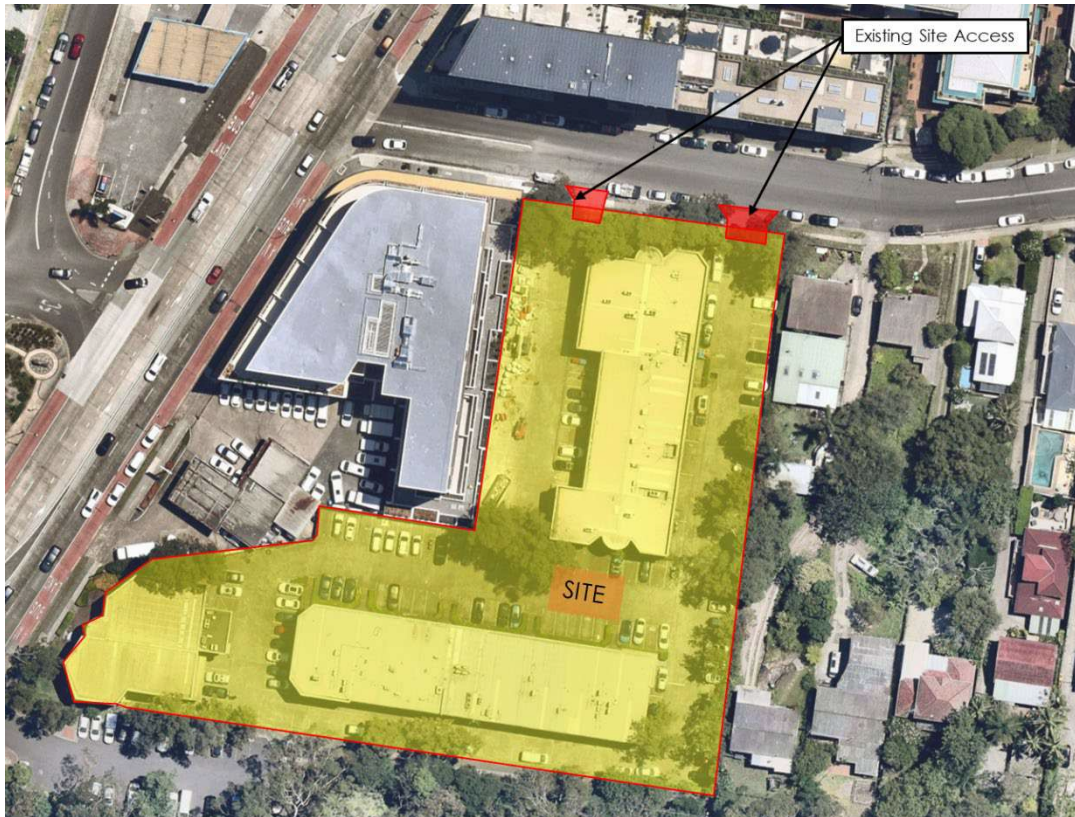
Figure 3.1: Existing Access Driveway on Delmar Parade
