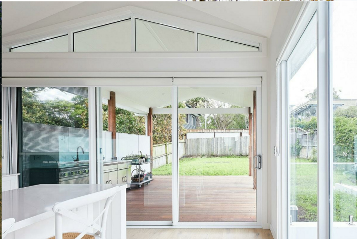
AL1 - Powdercoated aluminium windows and doors
