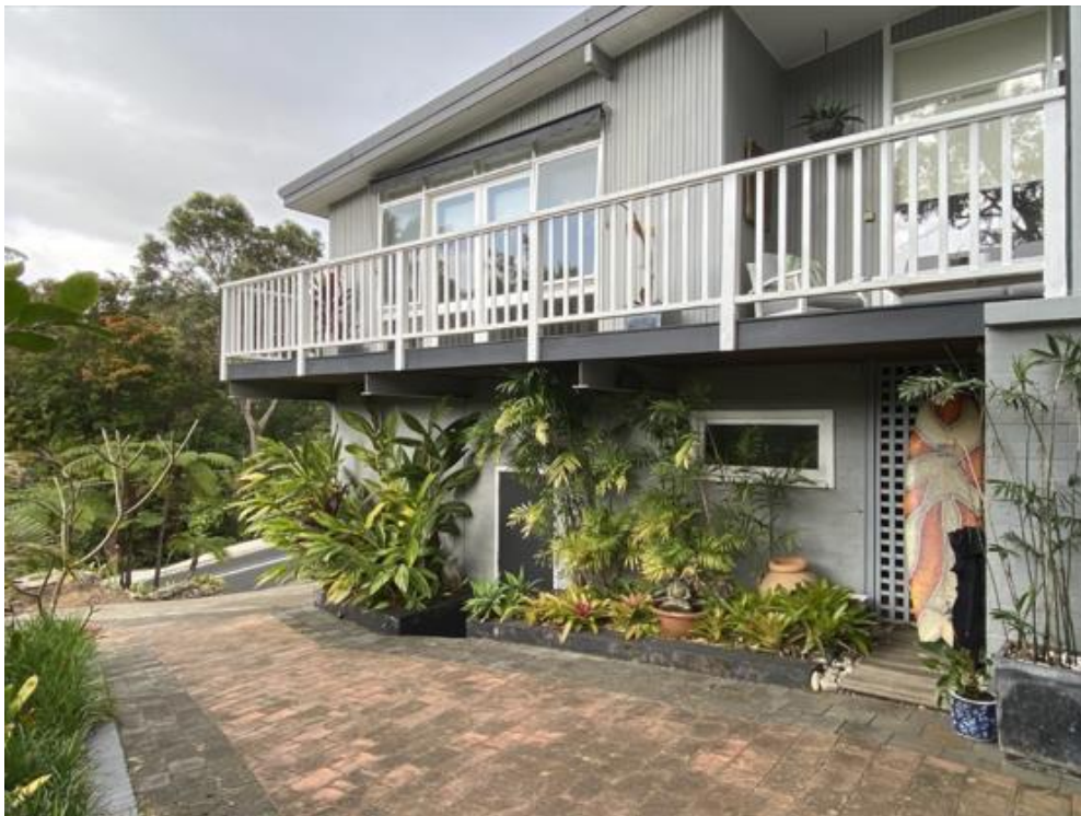
Figure 7. The existing balcony, looking south-west
