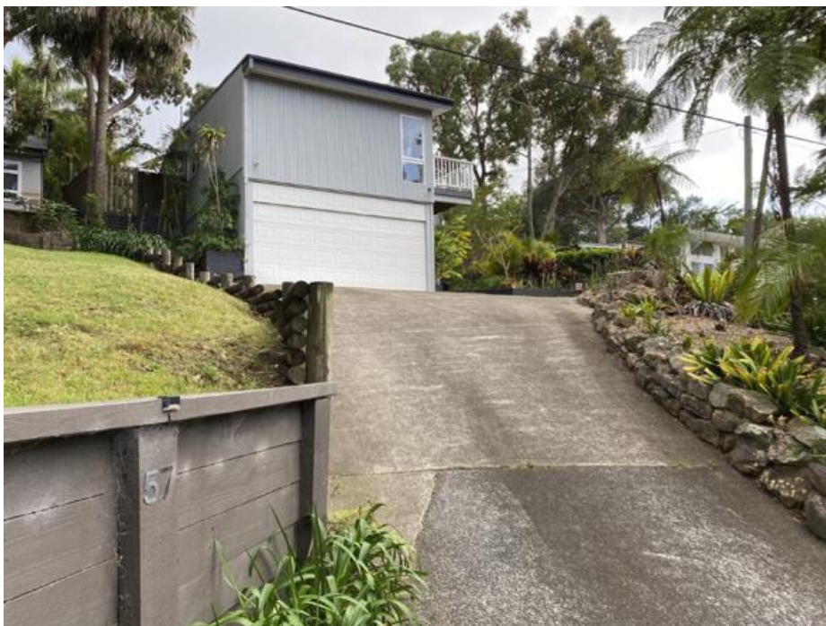
Figure 5. The dwelling façade, looking north
