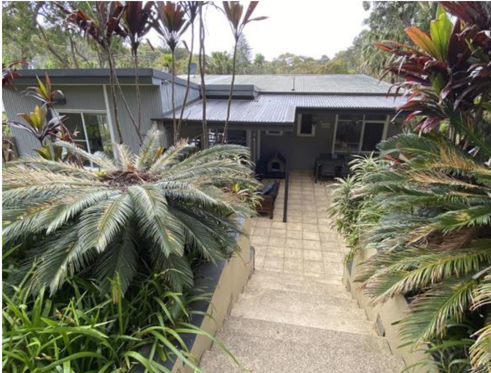
Figure 8. The rear of the dwelling, looking south
