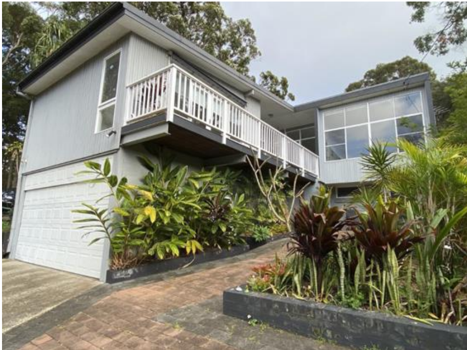
Figure 4. The subject site, looking north-west
