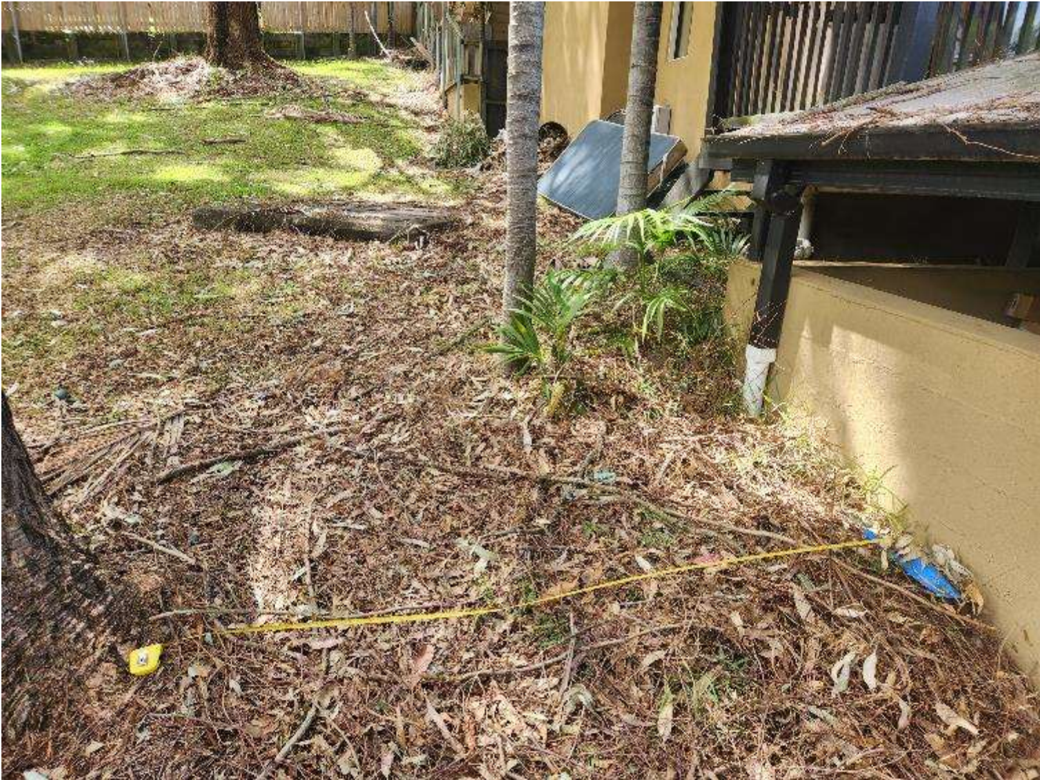
Fig. 13. Photo of tape measure from eave of the neighbour's car port to the buttress roots of T4.
