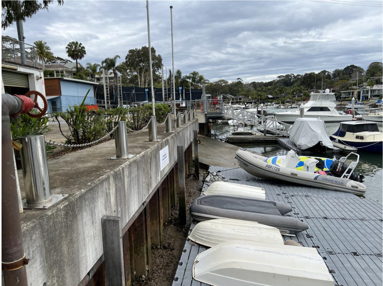
Figure 5: View of seawall at site on 12 August 2022, facing SSE
