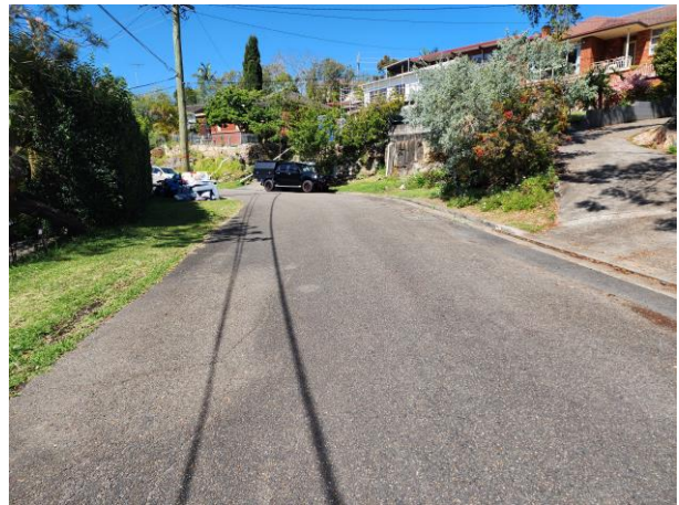
Sherwood Crescent, looking East
