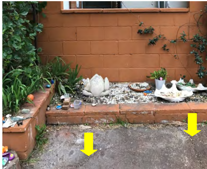
Photograph 4: Cracking in raised courtyard, looking west.
