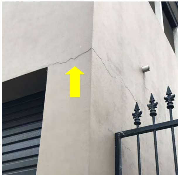
Photograph 5: Cracking observed in adjacent property (No. 33 Belgrave Street), looking west.
