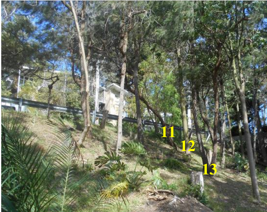
Figure 9 – showing the location of Trees 11 – 13 in the front setback of the subject property. Tree 11 has a severe tropism to the eastern quadrant.
