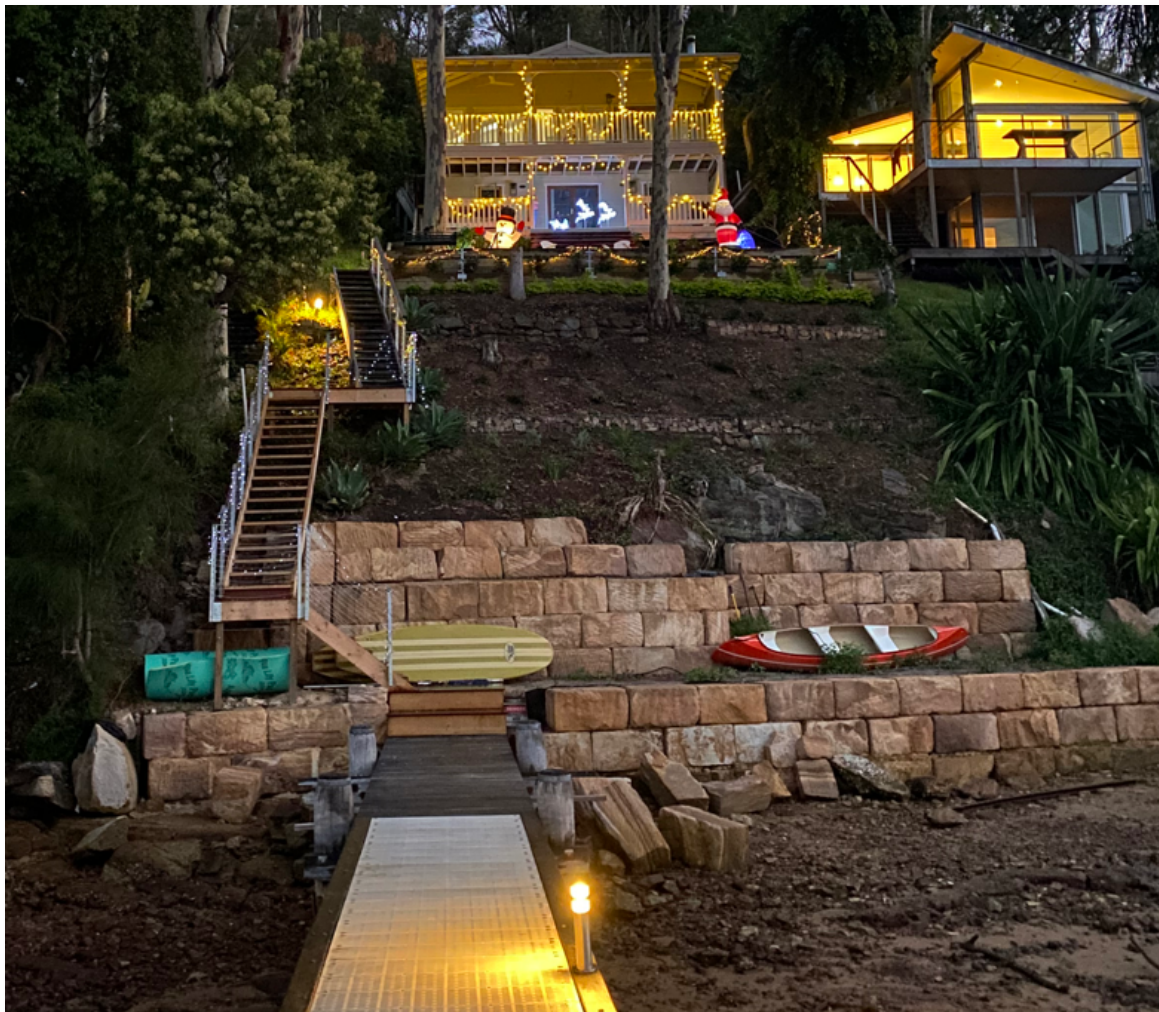
Figure 15 - Photograph of lower and upper tiers of the sea retaining wall, (taken prior to the ground failure)
