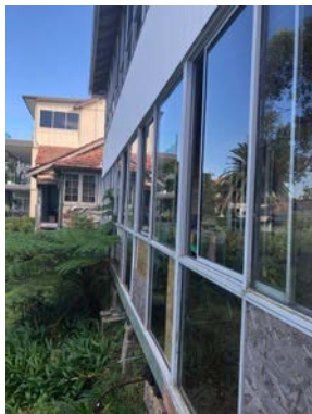
Figure 4.7 East side – Verandah Infill
