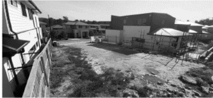
IMAGE 01 - SITE IMAGE OF THE REAR OF THE BLOCK
