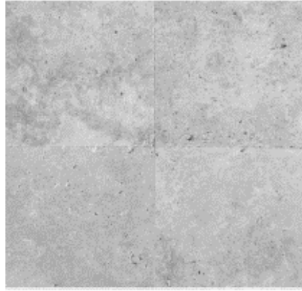
STONE PAVING - POOL SURROUND
