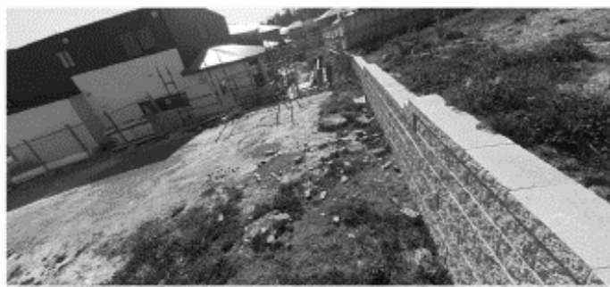
IMAGE 03 - SITE IMAGE OF THE REAR RETAINING WALL
