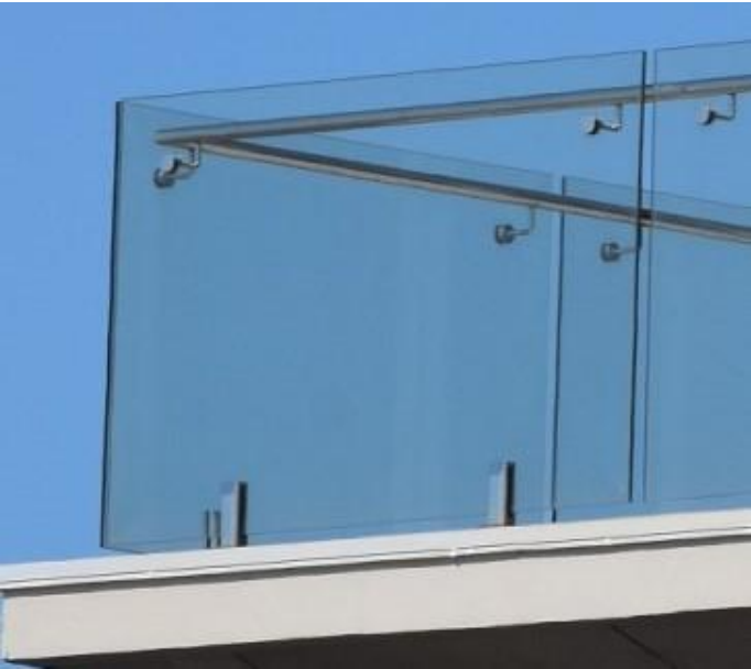
10 HR2 - Glass Balustrade WITH STEEL HANDRAILS
