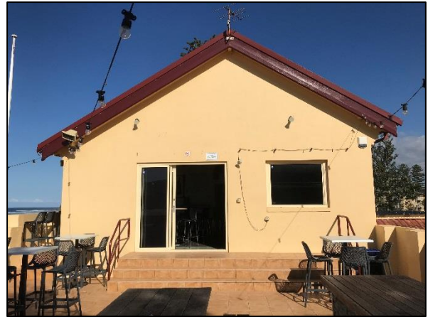
Figure 24. View of the Northern wing from the outdoor seating terrace.
