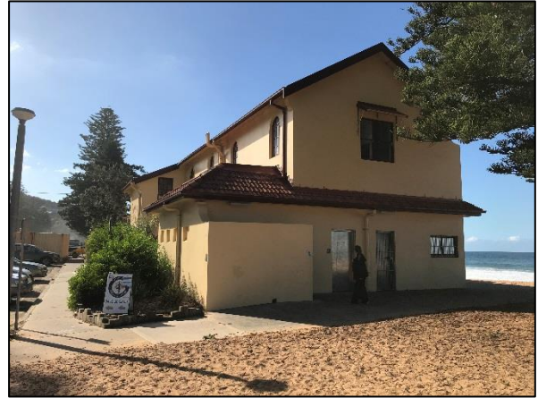
Figure 12. View of the southern wing and extension.
