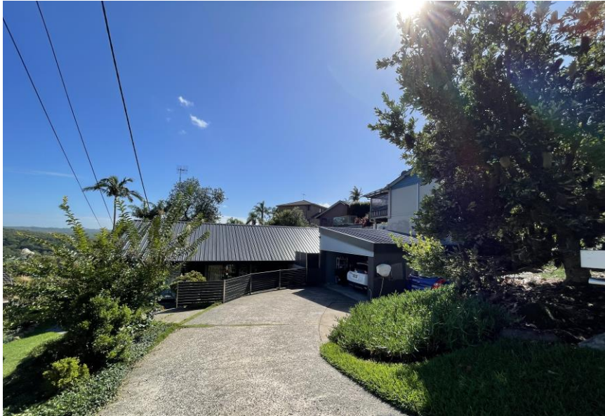
View of existing dwelling from street
