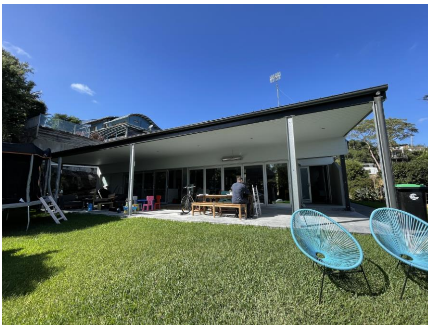
View of existing dwelling from the rear
