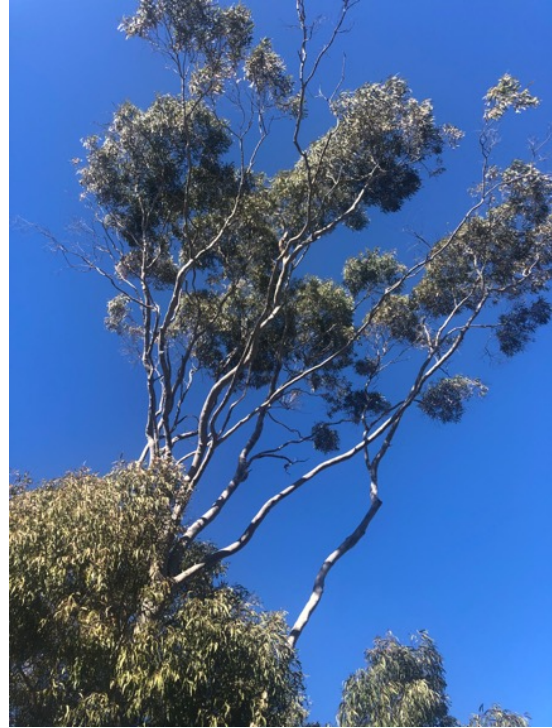
Figure 3 upper canopy of T1 displaying thinning canopy and twiggy dieback.
